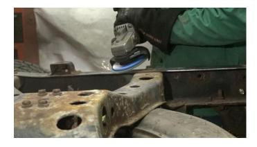
Clean the frame free of rust and debris, revealing bare metal.
